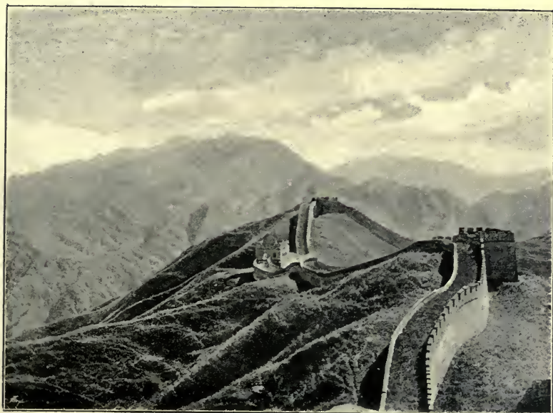
THE GREAT WALL OF CHINA.
